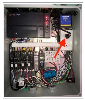
2) If your system includes an energy storage Automatic Transfer Switch (ATS), also unplug the black 12v DC battery backup lead in the lower ATS box.
